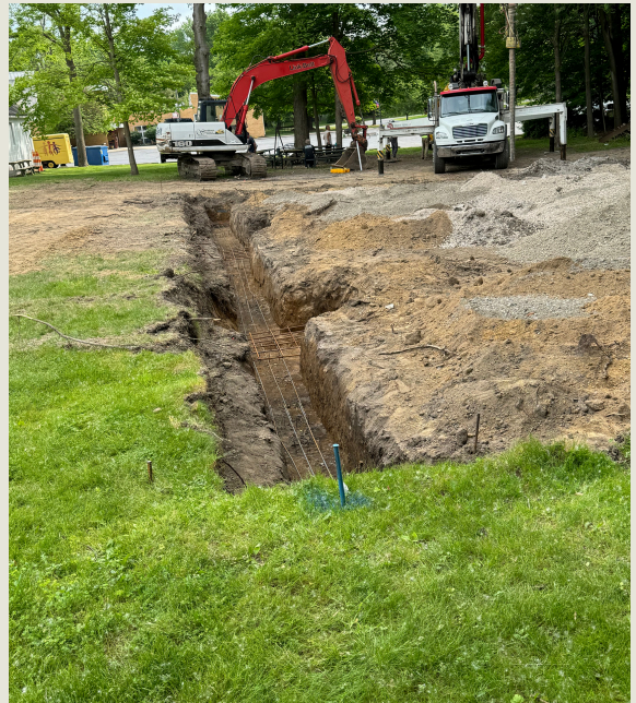
Ground Breaking & Pouring of the Footers
